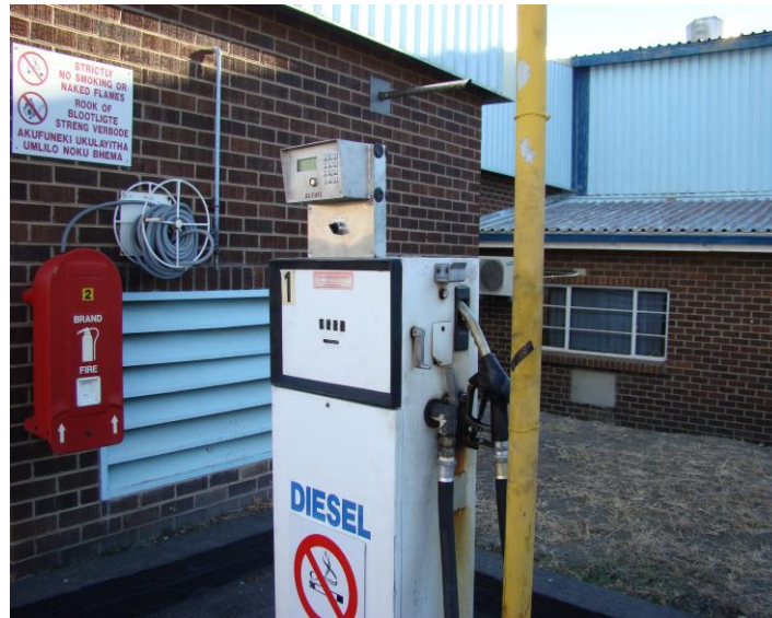
Figure 9 Image of the XL FUEL controller mounted on a mechanical pump
