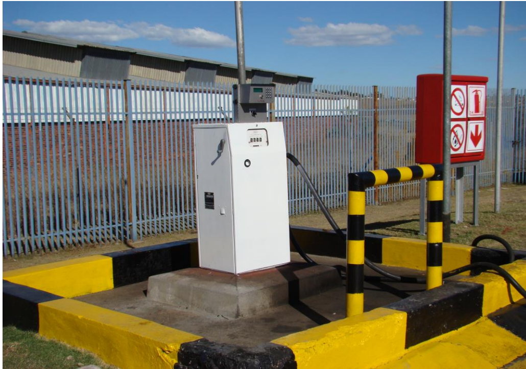
Figure 12 Image of the XL FUEL controller mounted on a very old mechanical pump
