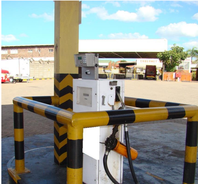
Figure 11 Image of the XL FUEL controller mounted on a mechanical pump
